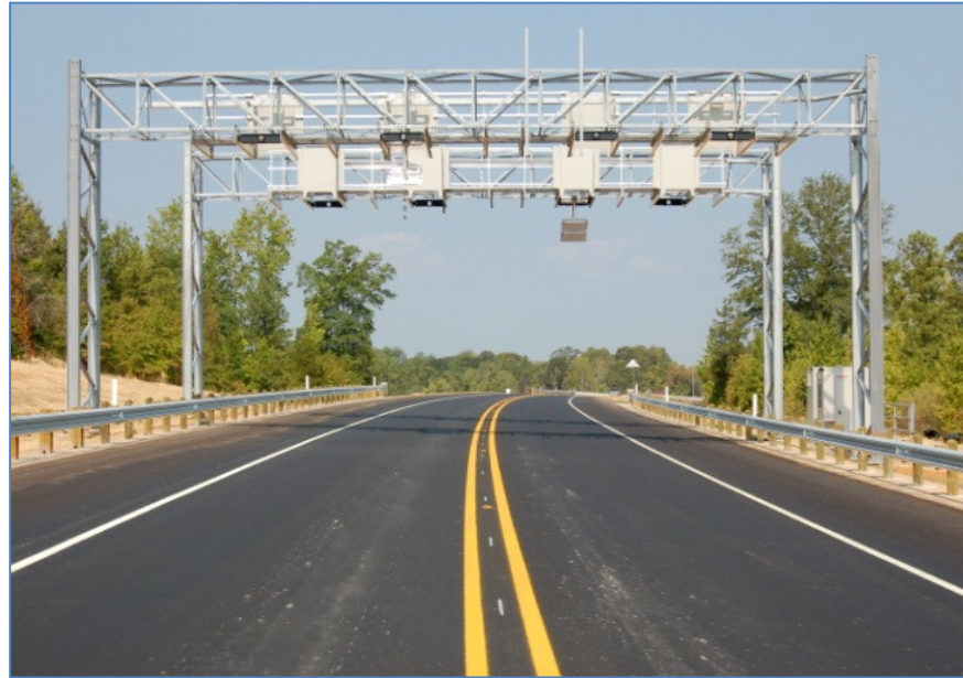
Figure 1: Example of an AET Toll Collection Point
